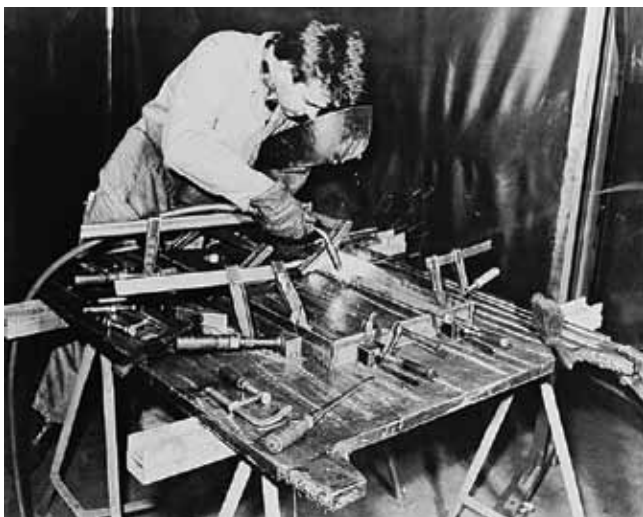
Figure 1. A "tack" table is a steel plate that has been ground flat that rests on its own legs or on saw horses. The locations for the stops are scribed on the surface and then the stops are tack welded. When the job is finished, the stops are broken free and the surface is cleaned with a hand grinder.
