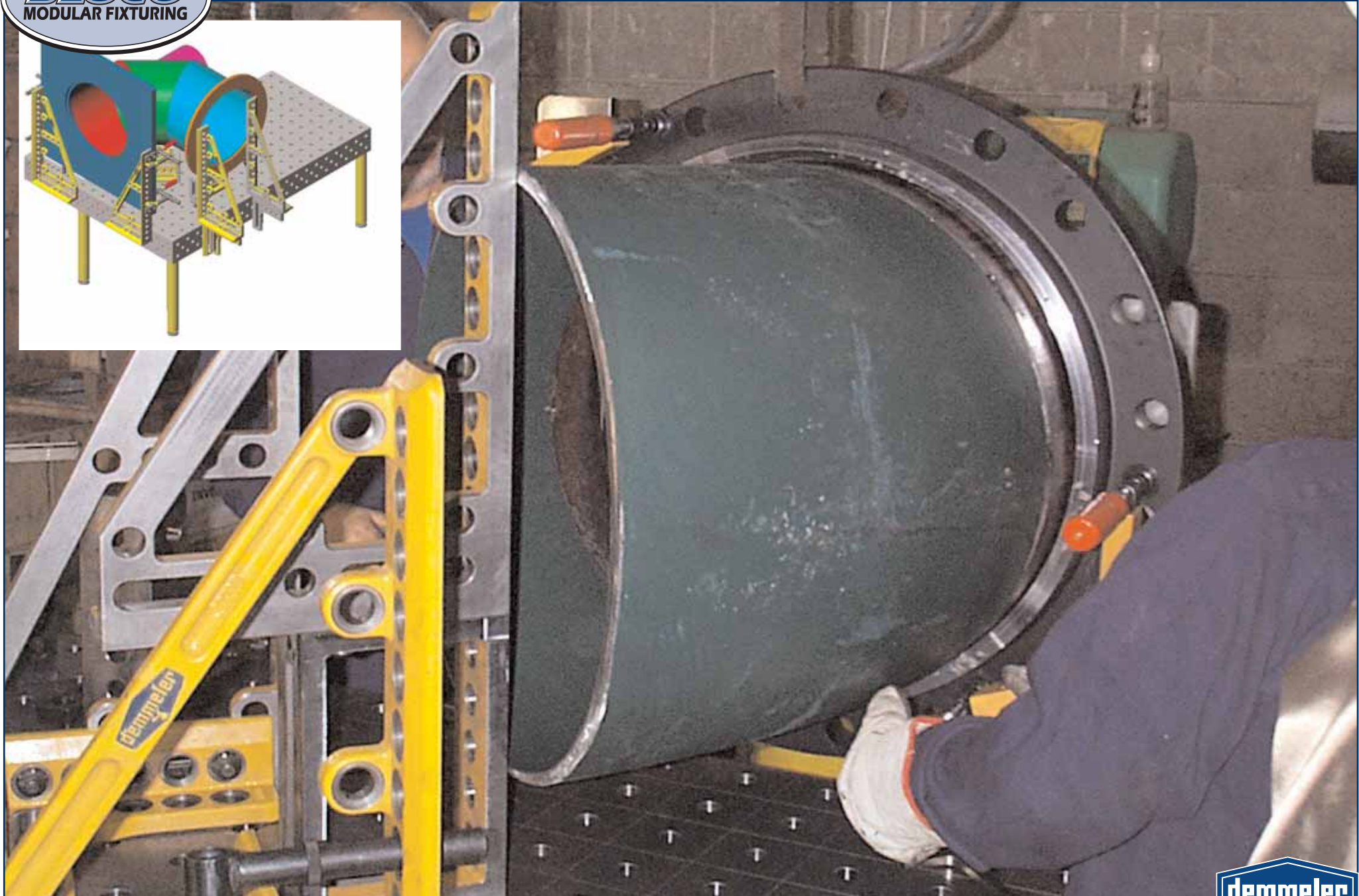
Large, 45 degree pipe squared to flange using large angles and clamps
